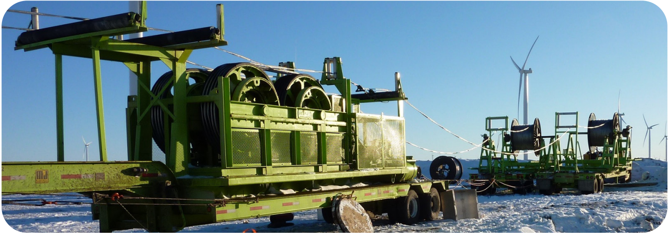
Figure 4: Payoff and bullwheel setup.
