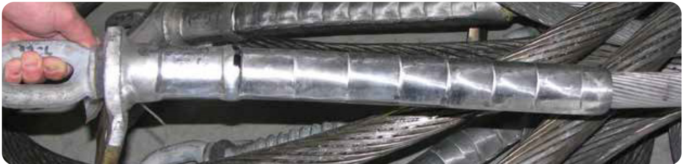
Figure 14: Compression dead-end.
