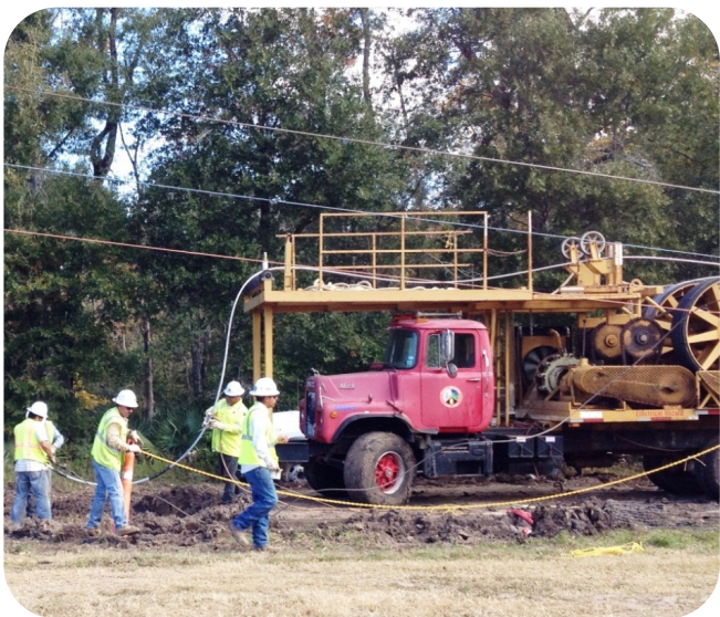
Figure 4: It is OK to drape slack conductor across a small roller. This would not be acceptable if the conductor was under tension or if the crew was pulling the tail to install a fitting.
