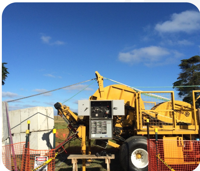
Figure 1: Example of a situation where bending is excessive even for ACSR. In this case, the payout reel is located downslope from the bull wheel, and the conductor bending angle is 35° around a four (4) inch roller. Photo courtesy of Trans Power New Zealand.
