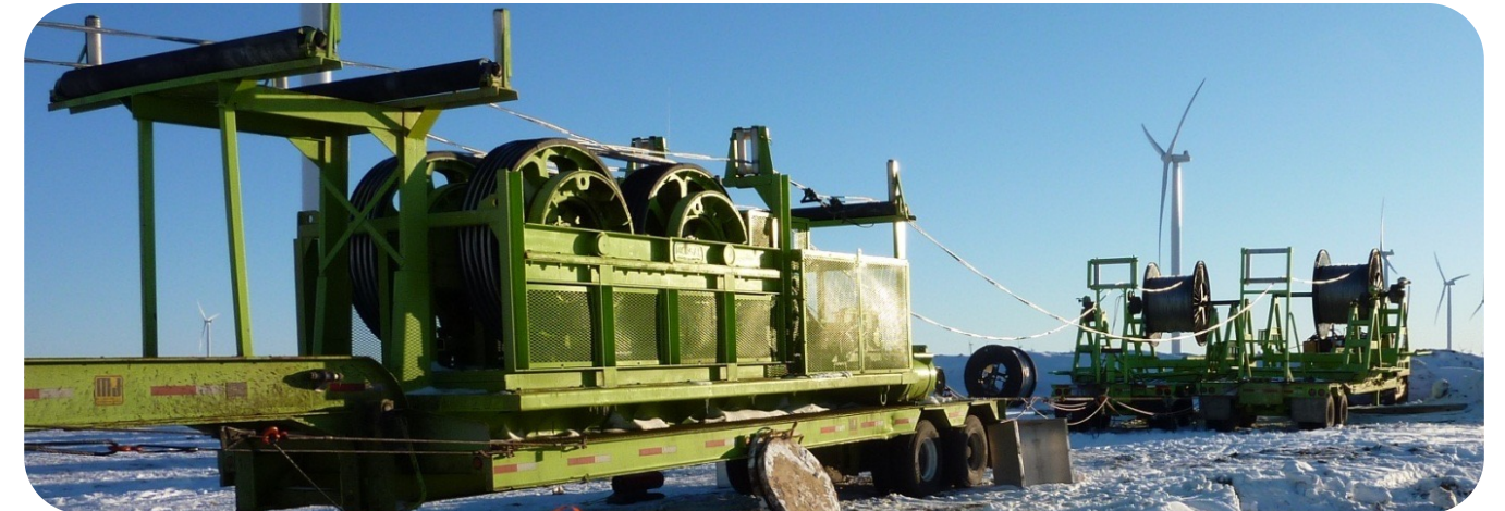
Figure 8: Payoff and bullwheel setup.
